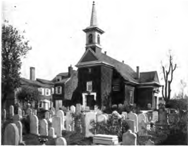
"GLORIA DEI," OLD SWEDES' CHURCH, SWANSON STREET, BUILT 1700
